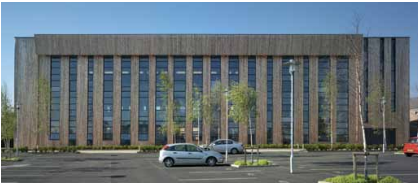
The Woodland Trust has a solid, cross-laminated timber structure, with external wood-fibre insulation and larch cladding
