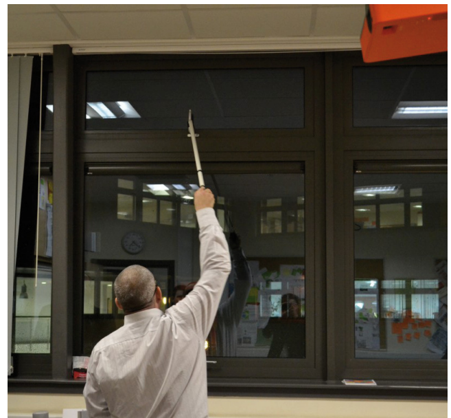
Figure 3.2 - Typical classroom window showing the openable top pane and bottom pane as well as the opening pole being used
