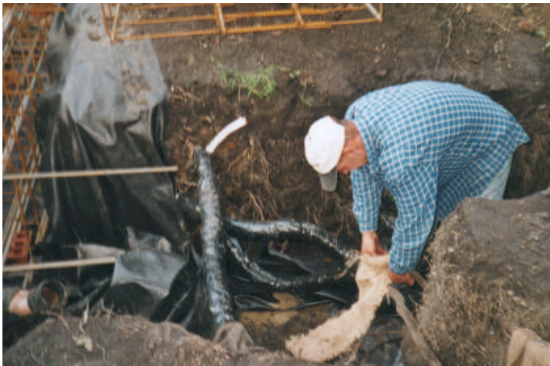
Tree roots had to be protected during the construction work
