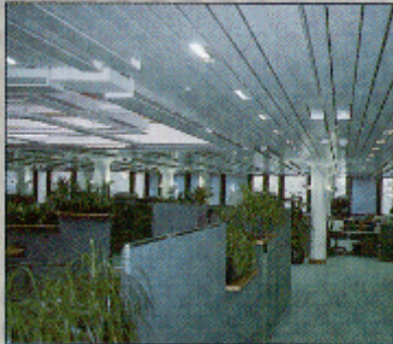
The open-plan offices, with the rooflight in the foreground. The rooflight gives little sense of light and space to the large ground floor office, partly because the plane of the downstand baffles is maintained.
