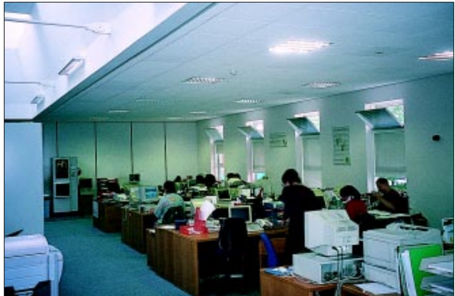
The glare from sun and sky is disappointing in view of the care devoted to the window system. This is due to diagonal sunshine coming past the ends of the light shelves, and bright spots on the blinds in bright sunshine.
