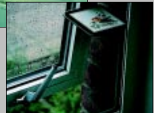
...the use of a coaster as a wedge. Gear hinges need friction to work.
